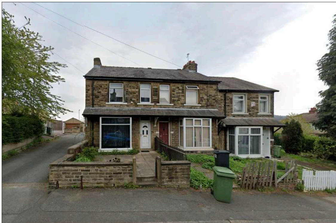
View of the existing three terraced dwellings on North Street adjacent to the site.
