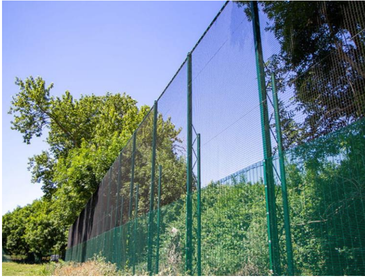
Figure 11: Example of weldmesh fencing with ball stop netting topper.
