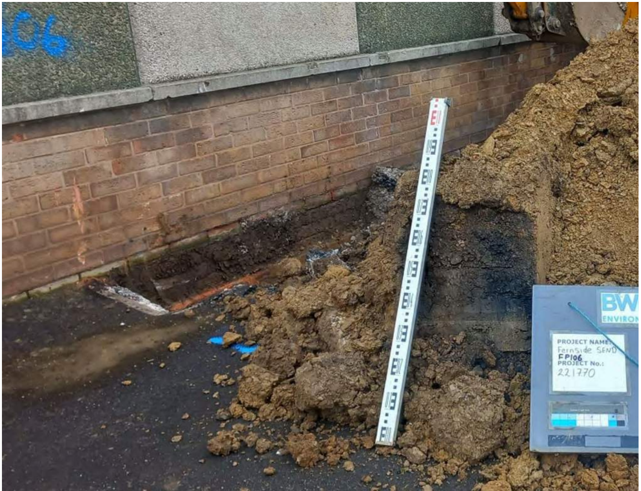
24/02/22 Photo 12 Looking Northwest. FP105 wrongly labelled 106. Note dark layer on arisings is top of buried former soil from 1.8m depth.
