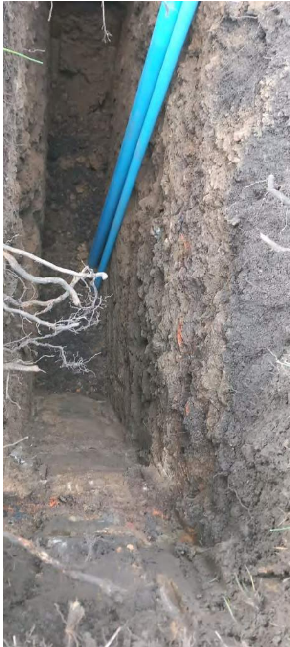
24/02/26 Photo 31 SA204. width 600mm x length 2100mm Topsoil 0.4m over made ground reworked natural with some brick to 1.1m over subsoil? To 2.0m over laminated siltstone bedrock.
