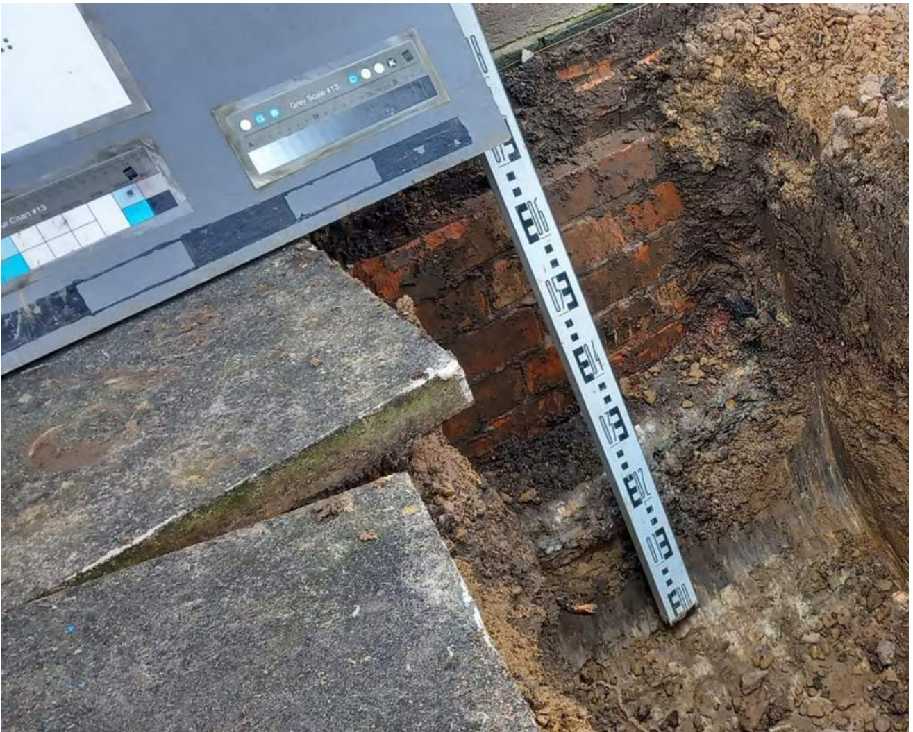
24/02/22 Photo 14 Looking West. FP101. Strip Footing at 0.5m depth on bedrock.
