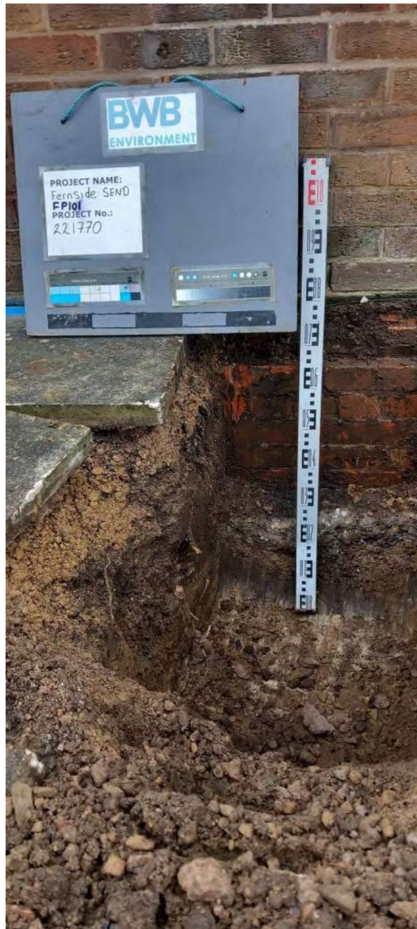
24/02/22 Photo 15 Looking West. FP101. Strip Footing at 0.5m depth on bedrock. 2" Paving flags over limestone aggregate over gravelly clay backfill to 0.5m.
