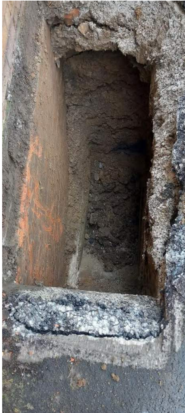
24/02/22 Photo 11 Looking ESE. Concrete footing at 1.7m depth below loose backfill.
