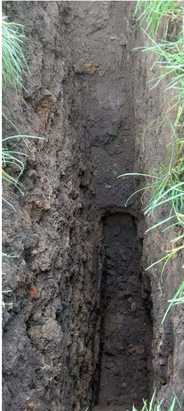
24/02/26 Photo 33 SA203. width 600mm x length 2100mm Topsoil 0.4m over made ground reworked natural with some brick to 1m over subsoil? To 2.9m
