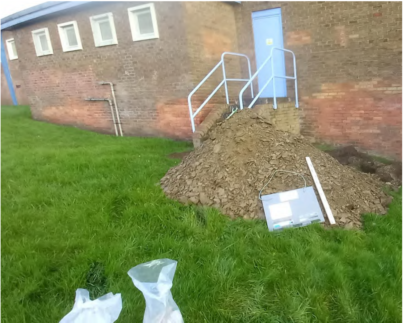
24/02/23 Photo 17 TP203. Moved due to drainage services. Adjacent to swimming pool.
