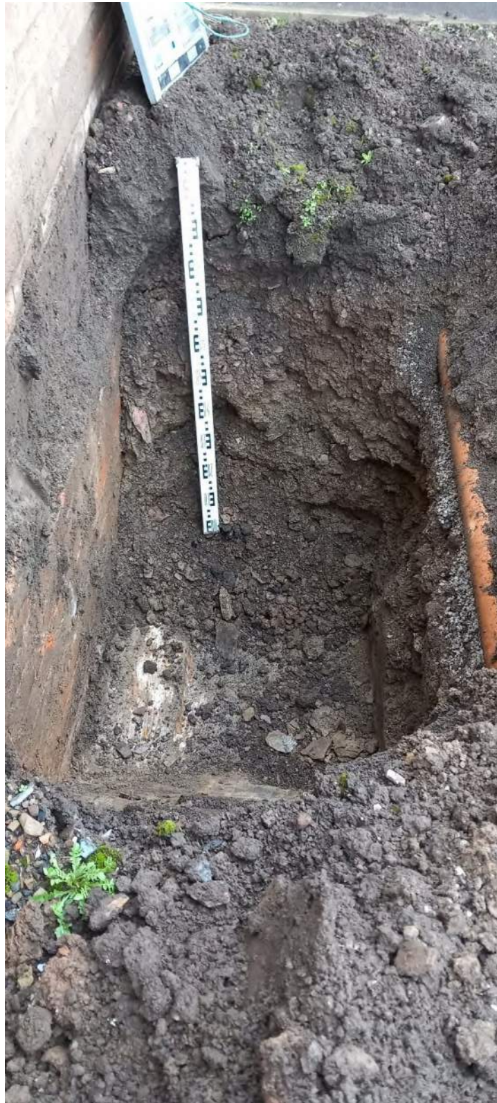
24/02/22 Photo 5 Looking ESE. FP103. 0.5m topsoil over Loose Made ground backfill. Footing at 1.1m
