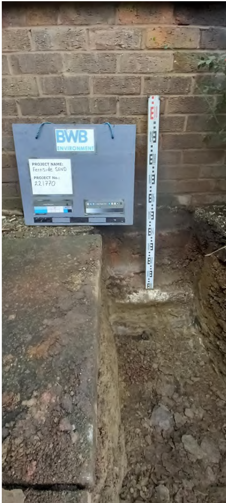
24/02/22 Photo 1 FP102. Looking East. Concrete strip footing at 0.45m depth. On bedrock.
