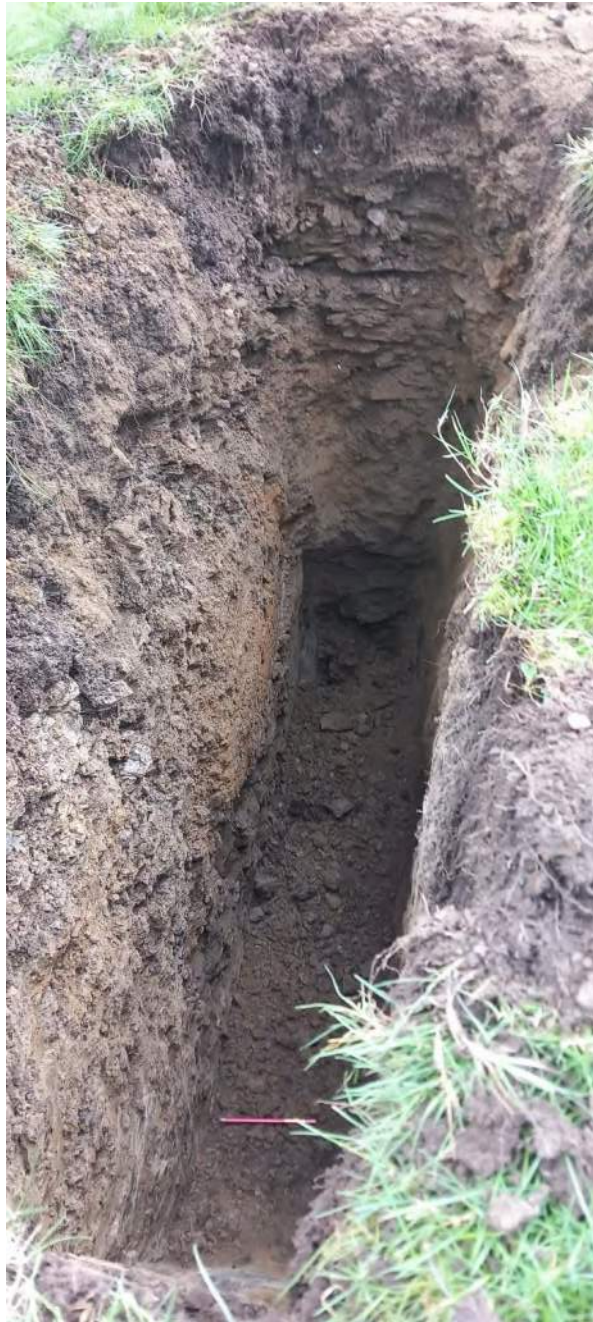
24/02/26 Photo 37 SA202. width 600mm x length 1800mm Topsoil 0.3m over subsoil to 0.4m over laminated siltstone bedrock to 1.5m.
