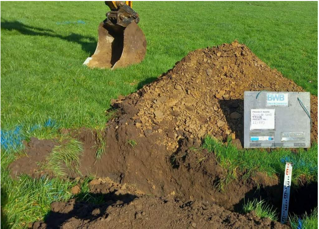
24/02/23 Photo 24 TP202. Topsoil 0.35m over Stiff gravelly Clay subsoil over weathered laminated siltstone bedrock at 0.95m
