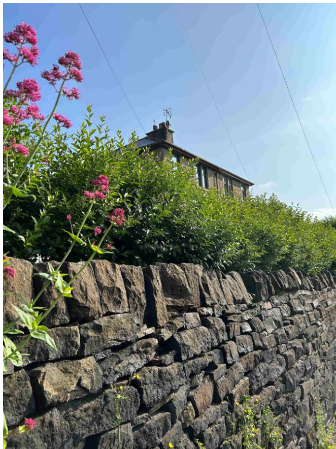
Image 3 – View of No.8 from the Greenfield Road pavement, note the roof planes are barely visible.
