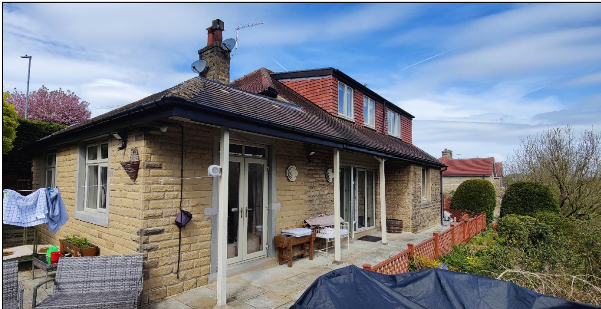
Photograph of the existing rear elevation
