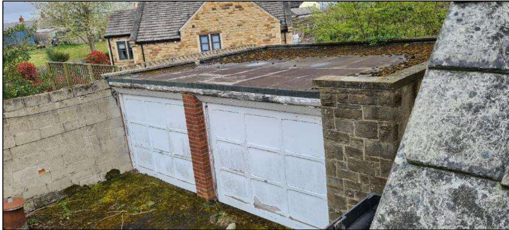
Plate 5. The garage viewed from the steps of the adjacent dwelling
