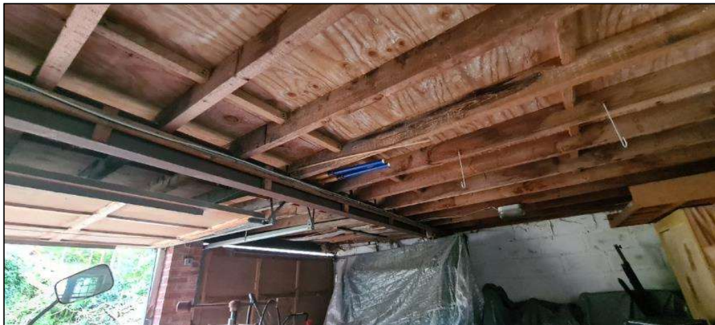
Plate 6. The interior of the garage roof
