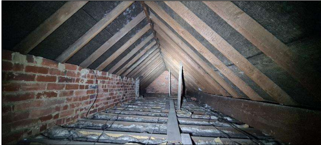
Plate 3. The roof void in the apex of the pitched roof
