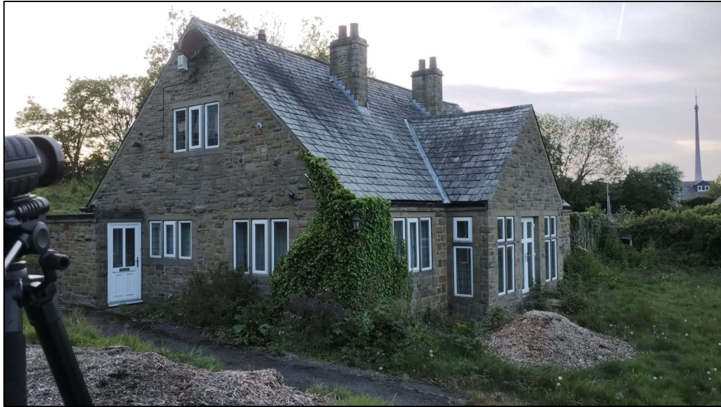
Plate 8. Bungalow viewed from surveyor Position 2 on 6 th May 2025
