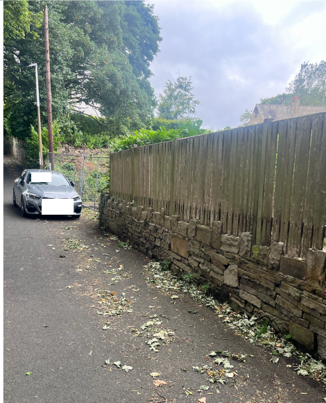
Figure 9 – Telegraph Pole (TP) and Lamp Post (LP) and 3 rd party fence at the existing access ( Source; Private Photo 26/8/24).
