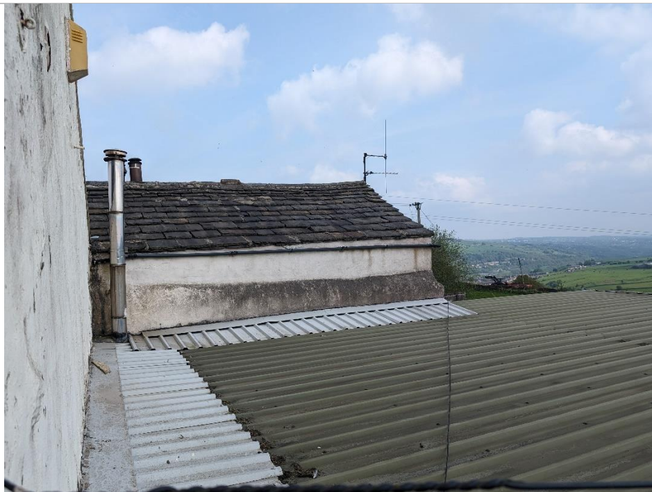
Photo 6. View of dwelling roof and garage roof.
