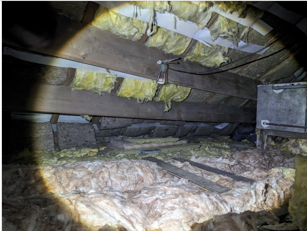
Photo 10. Loft of dwelling.
