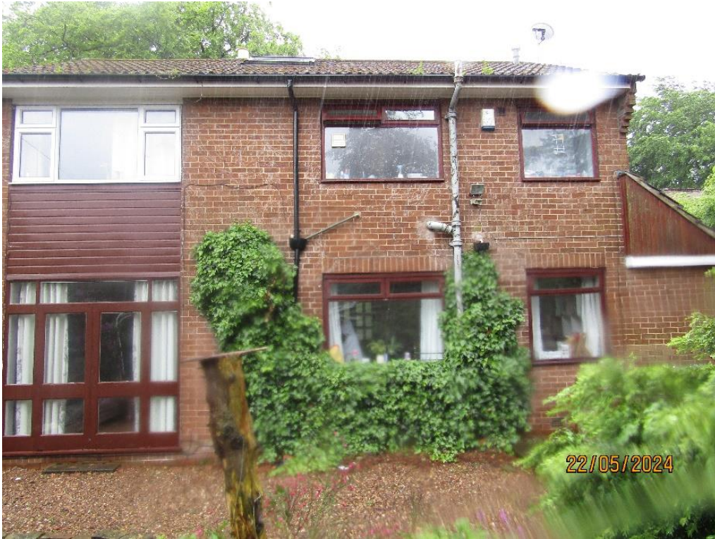
Image 5. Rear view of property
