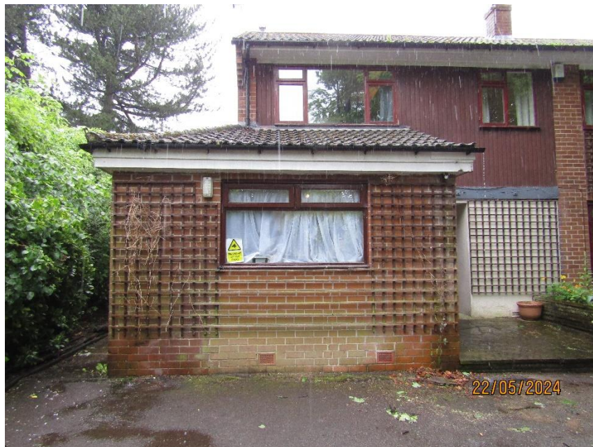
Image 2. Front elevation showing existing single storey extension
