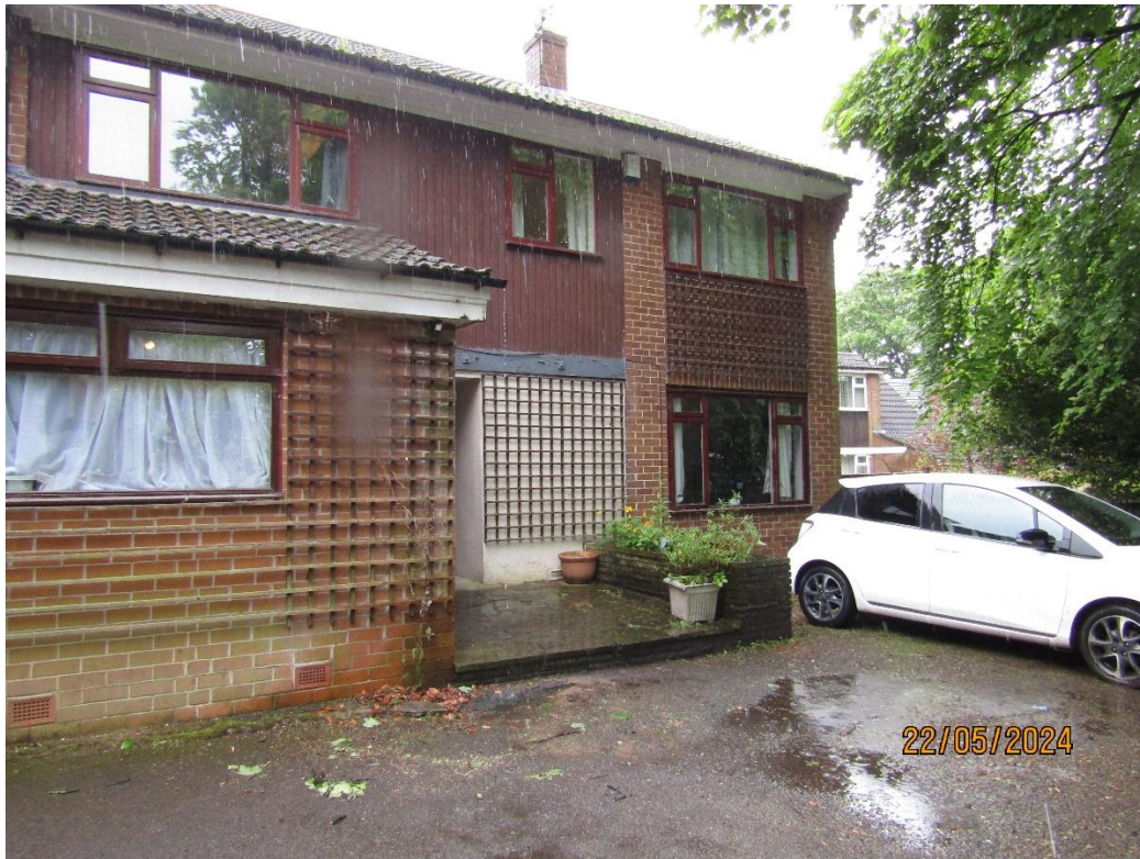
Image 1. Front elevation of property
