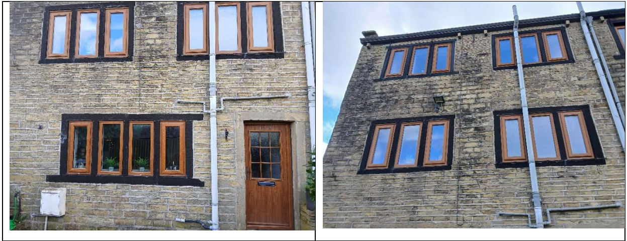
Figure 3: Rear elevation of No.132 (ground, first and second floor).
