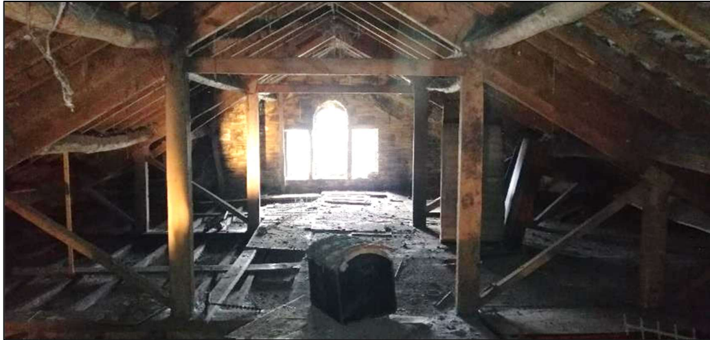
Plate 9. Roof-space of B1
