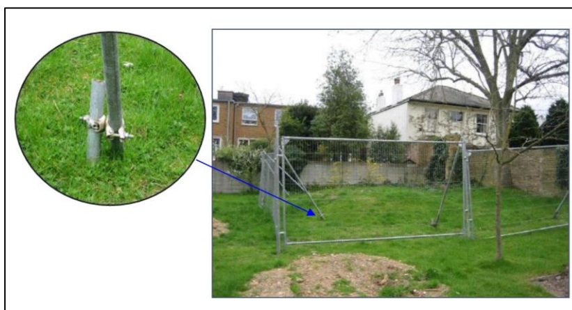
Figure 2.1: Example of mesh welded type barriers in-situ.
