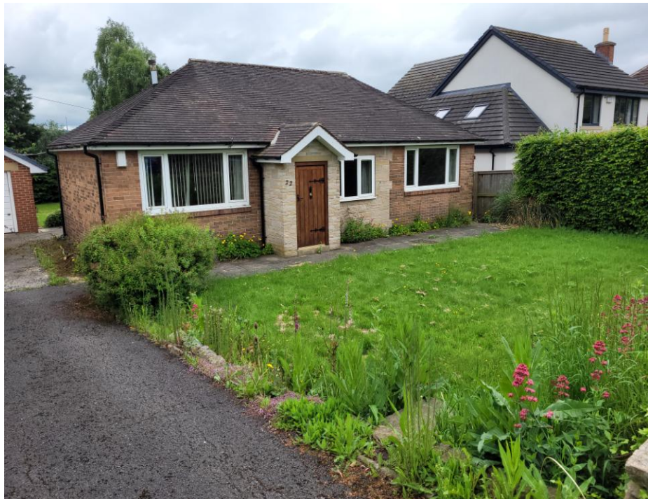
View of front of property
