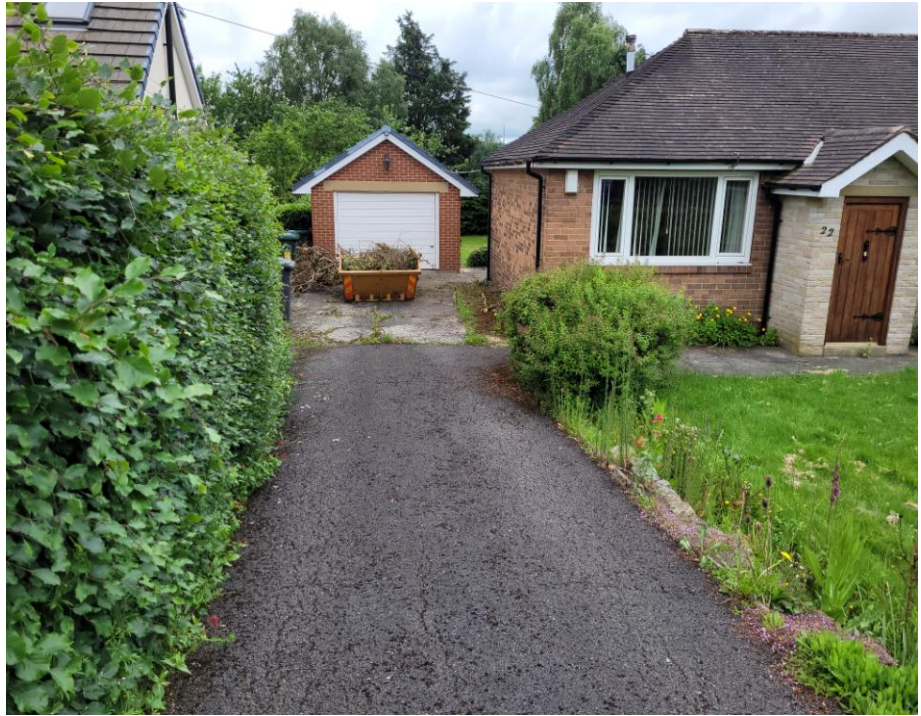
View of front of property
