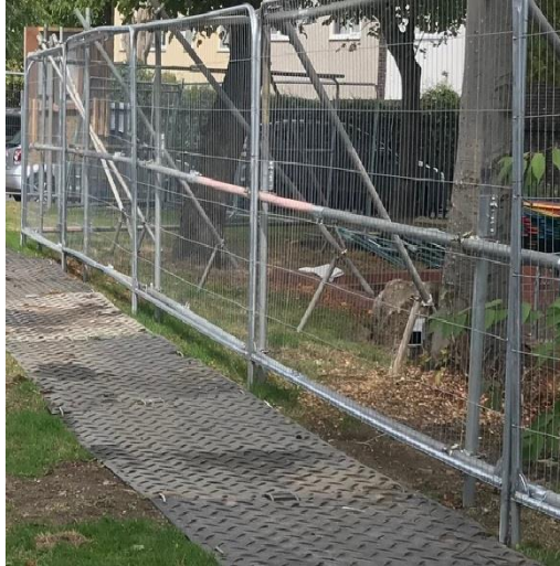
Picture 2. Displays a combination of Tree Protecting Fencing & Ground Protection
