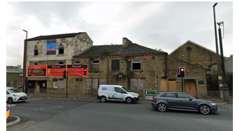
IMAGE SHOWING CONDITION OF BUILDING
