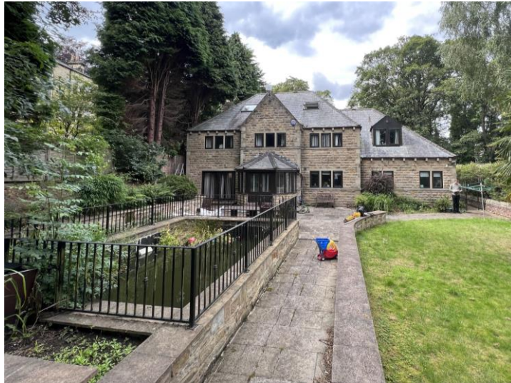
Rear of Dwelling, Site Survey
