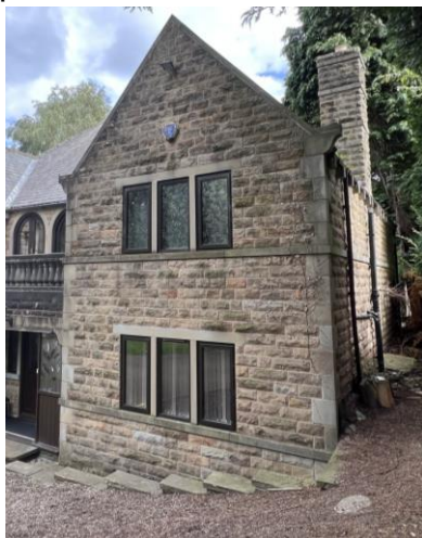
Stone Heads, Cills, Mullions and Quoins Shown on Front and Rear External Walls
