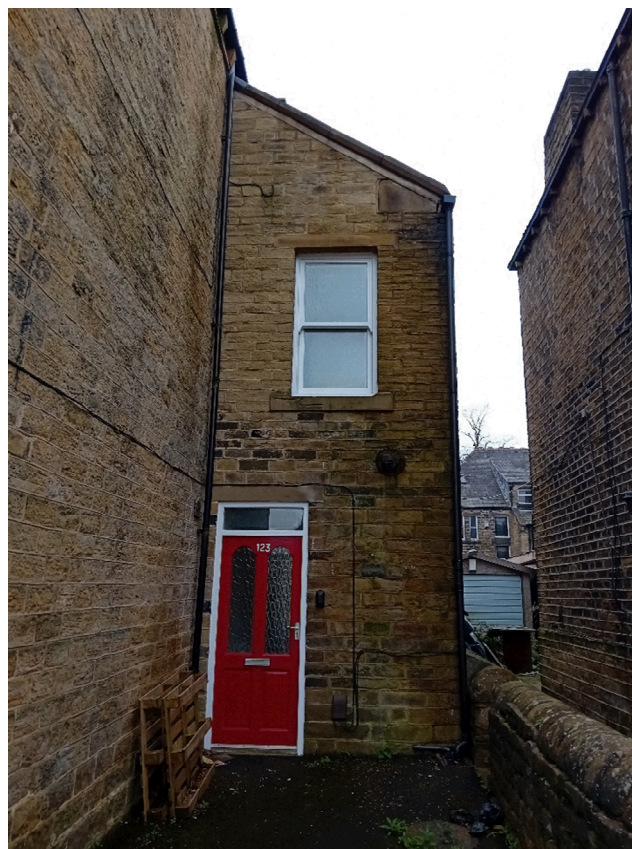
Fig 5. Front elevation of 123 Trinity Street.
