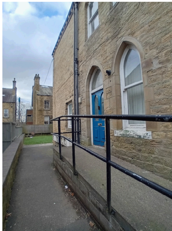
Fig 3. Left hand side elevation and entrance to 119 Trinity Street.
