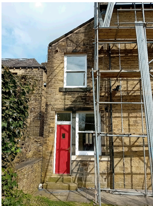
Fig 6. Rear elevation of 123 Trinity Street.
