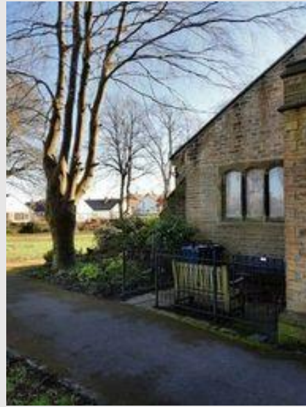
Plate 6: T010 and the existing church building/site of the proposed extension
