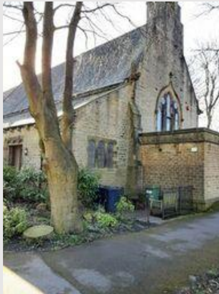
Plate 7: T010 and the existing church building/site of the proposed extension
