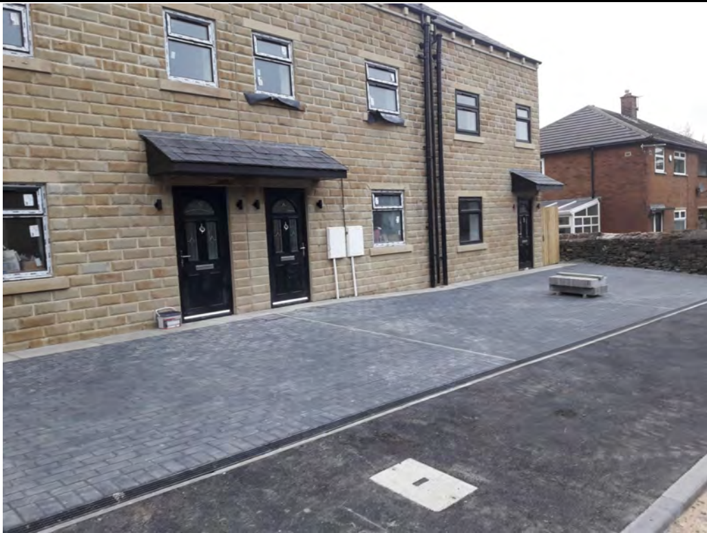
Photo 6: RGS Site Visit 01.05.24. Sufficient hard-standing placed at the front.
