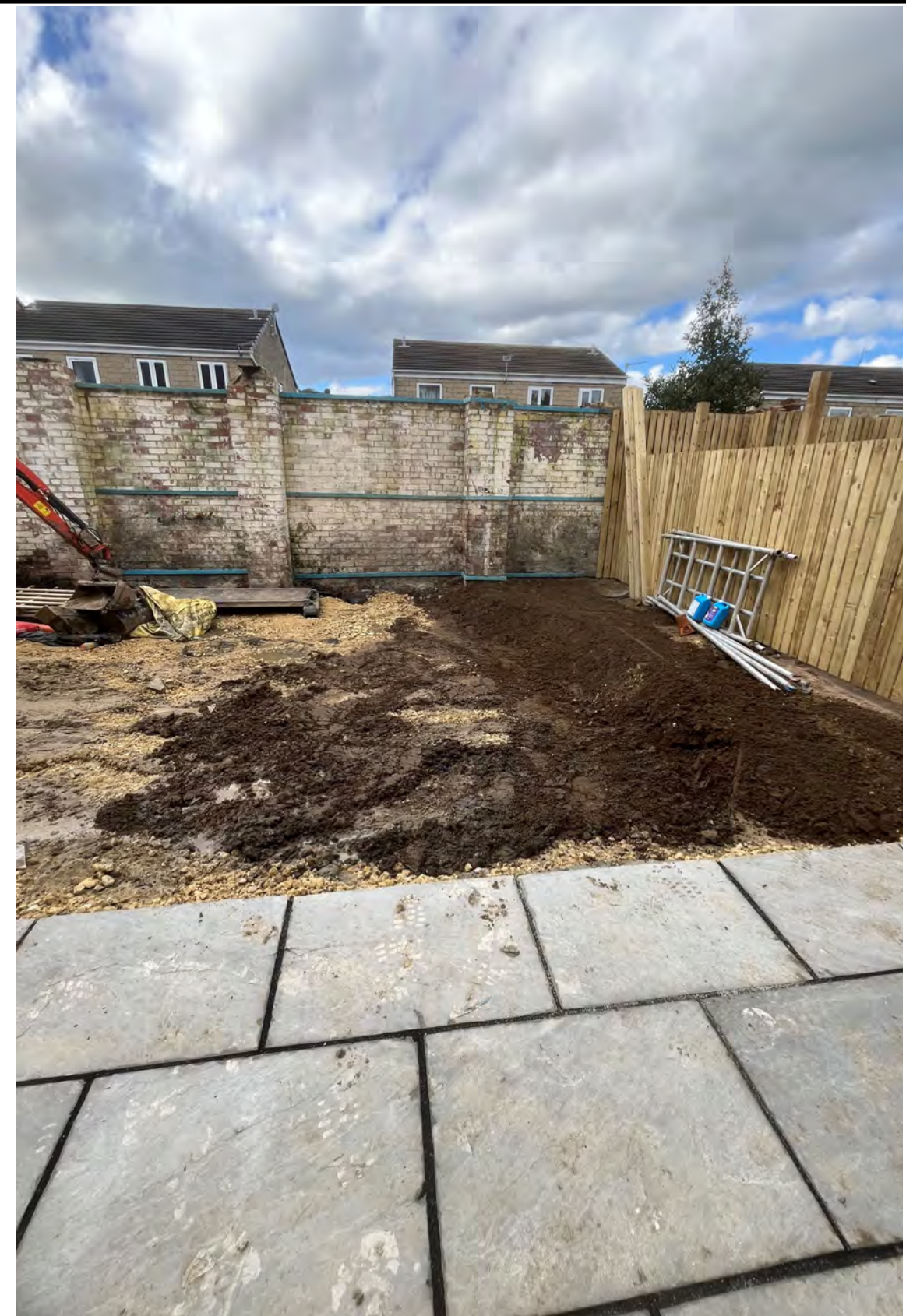
Photo 4: Client Photograph 17.04.24. Initial placement of topsoil above membrane and stone.
