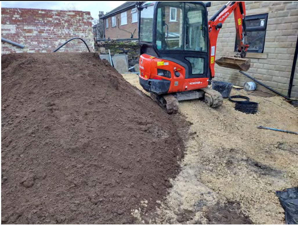
Photo 3: RGS Site Visit 27.03.24. Topsoil stockpile. Membrane and stone already being placed.
