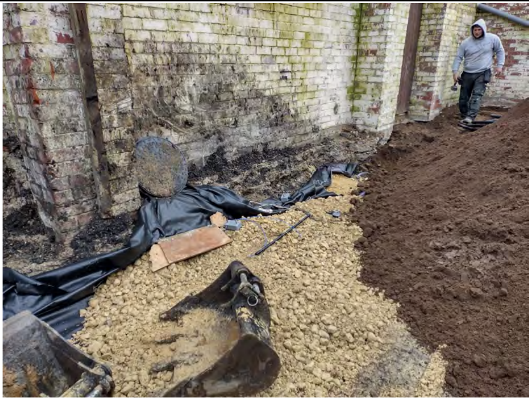
Photo 2: RGS Site Visit 27.03.24. Membrane placed and lapping at the sides.
