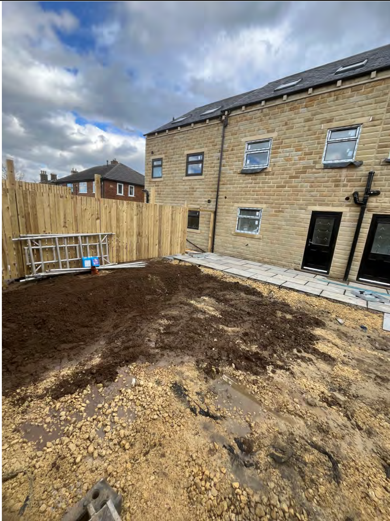
Photo 3: Client Photograph 17.04.24. Initial placement of topsoil above membrane and stone.
