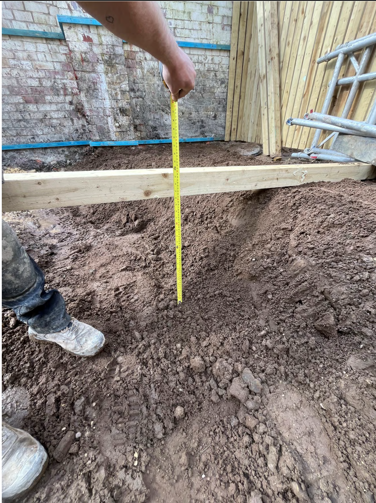
Photo 1: Client Photograph 17.04.24. Placement of topsoil above membrane and stone.
