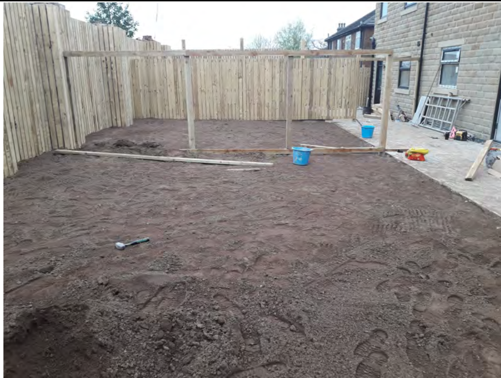
Photo 5: RGS Site Visit 01.05.24. Topsoil placed across all garden areas.
