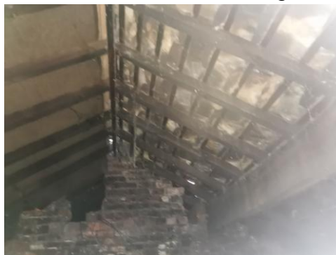
Photo 2. Interior of building.
