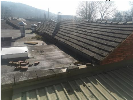
Photo 3. Roofs of building.
