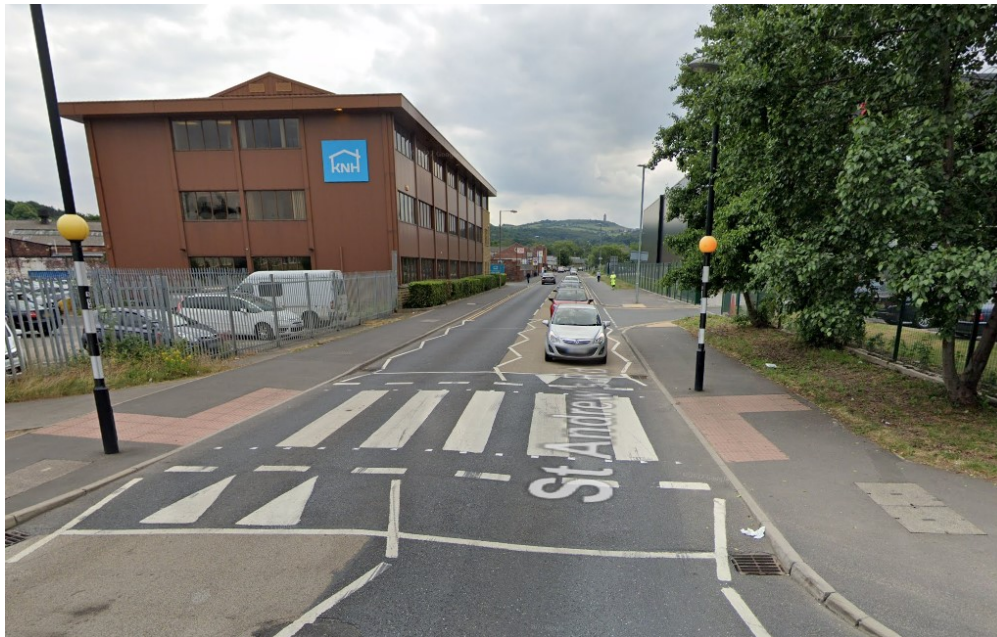
Image 1 - The Former Perseverance House from St Andrew's Road.
