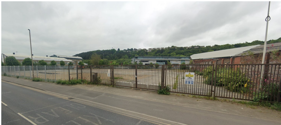
Image 4 - The Cleared Site as viewed from the South
