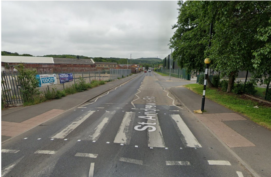
Image 3 - The Cleared Site as viewed from the North
