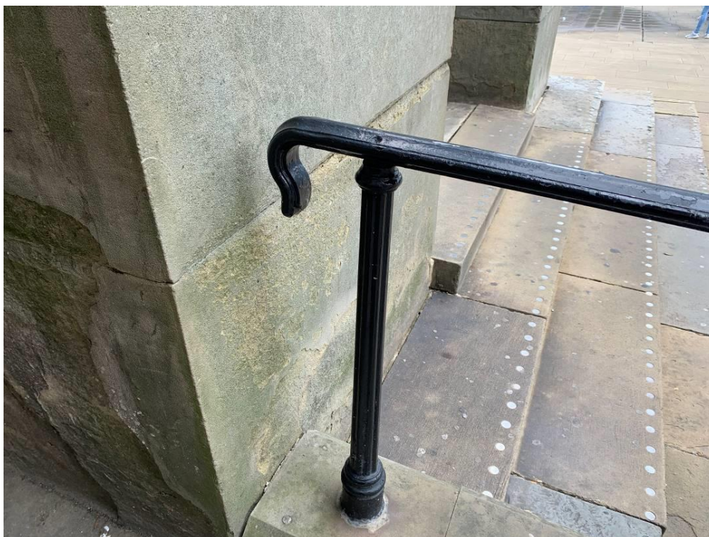
Photograph 9 – Handrail to ramped access
