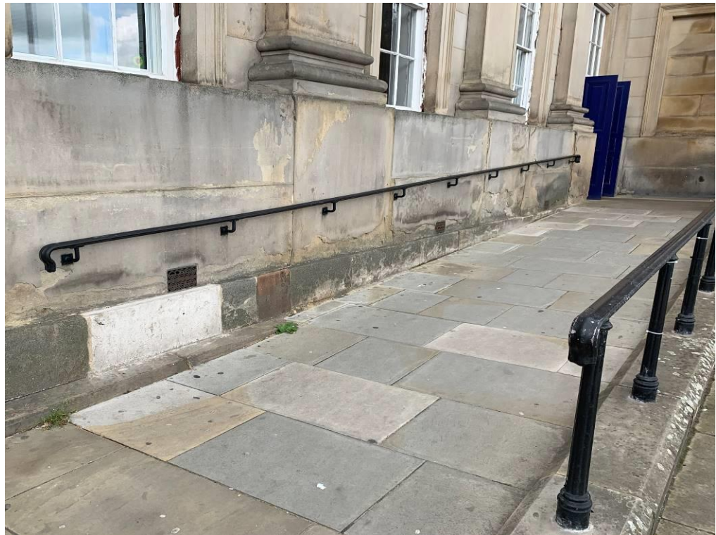
Image 10 – Existing handrail to ramped access
