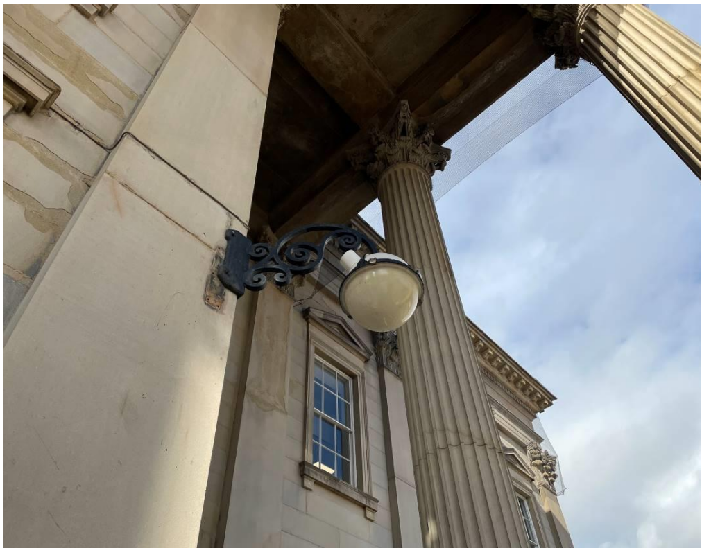
Photograph 8 – Existing globe lights to entrance
