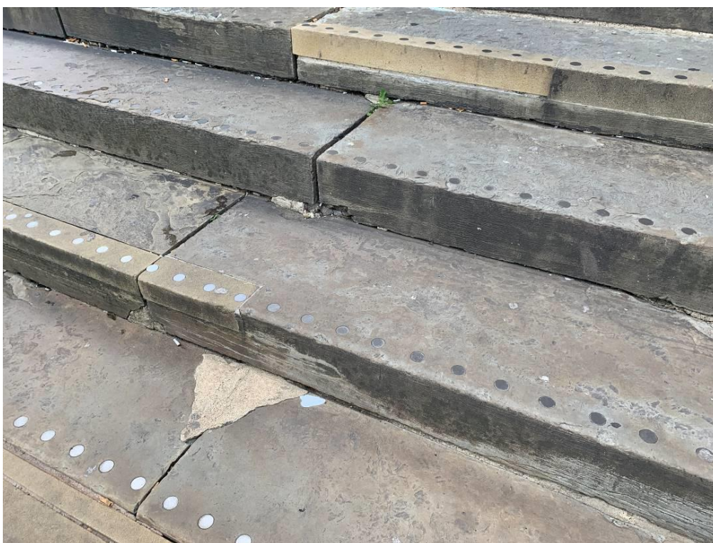
Photograph 10 – Areas of historic pointing repairs
