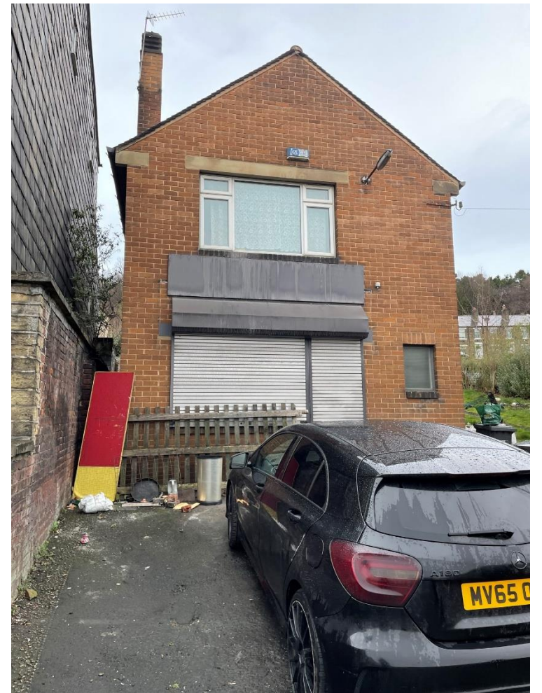
Existing 2-storey red brick building on site (to be demolished)
