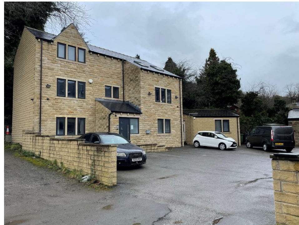
More contemporary 3-storey residential building to the west of the site
