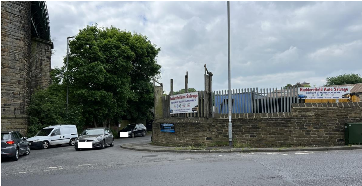
Fig 4: Site photo showing remnants of the support structures from the previous 1 x 48 sheet freestanding billboard at the Application Site of Huddersfield Auto Salvage, Paddock Foot Huddersfield, HD1 4RY
