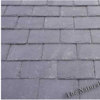
NATURAL BLUE SLATE ROOF COVERING
