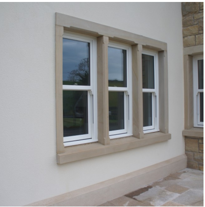
SILICONE THROUGH COLOUR RENDER WITH ASHLAR HEADS, CILLS AND MULLION
