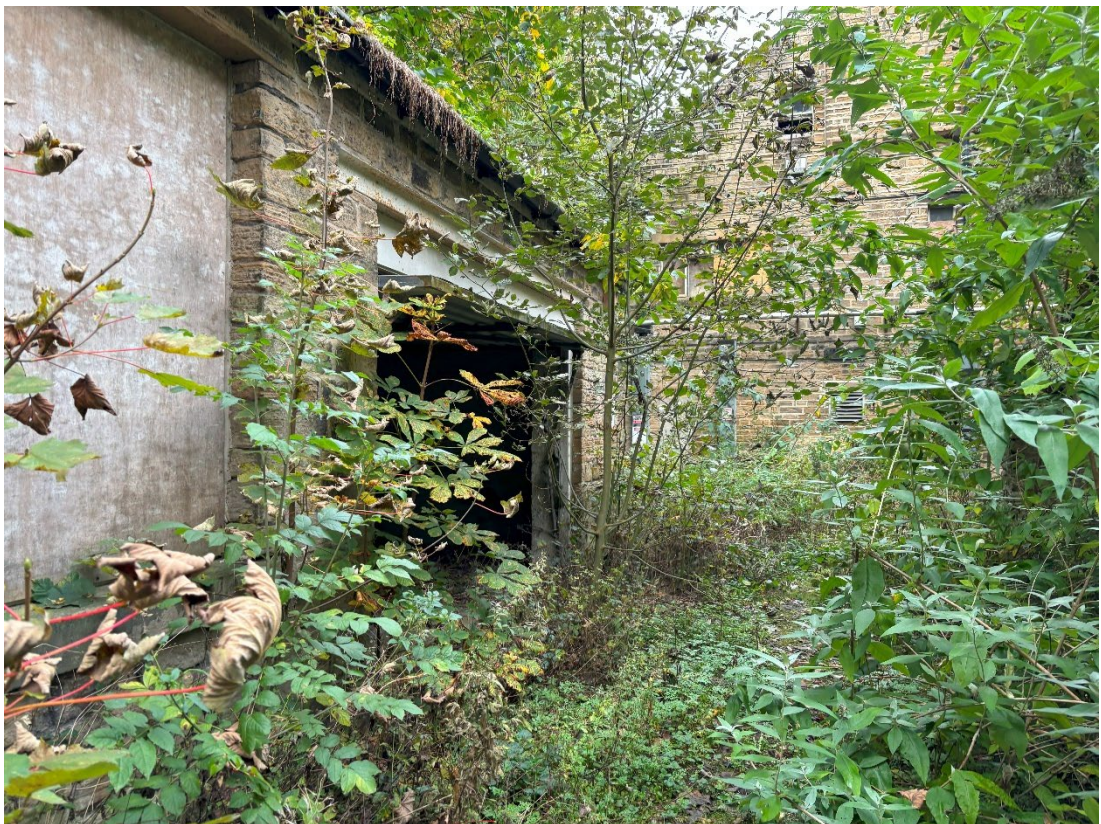
Photograph 20. Self-seeded trees and scrub was encroaching onto the Site.
