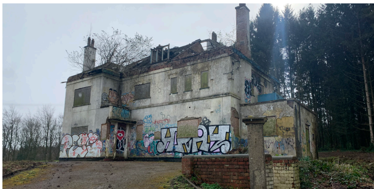
Existing vacant Dale Bank dwelling in Arts and Crafts style with chimneys.
