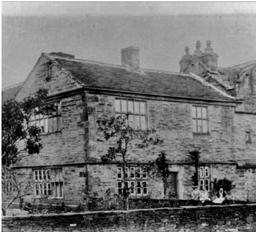
circa 19c (view from east) – Looking directly at what is now referred to as Kirkby Grange Hall. Note the original position of the front door, between the windows.
