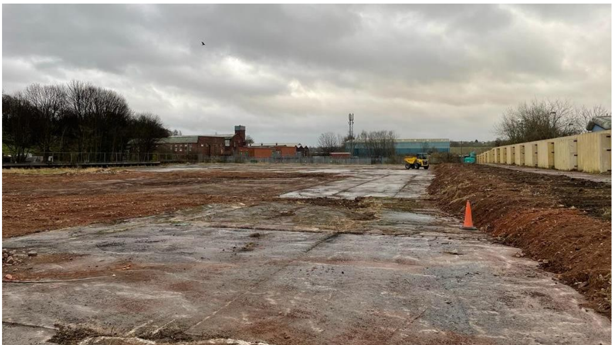
Figure 4 - Concrete ground surface with raised section and main operational area in background
