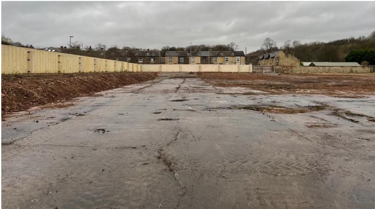
Figure 3 - Concrete ground surface with proposed access location in background
