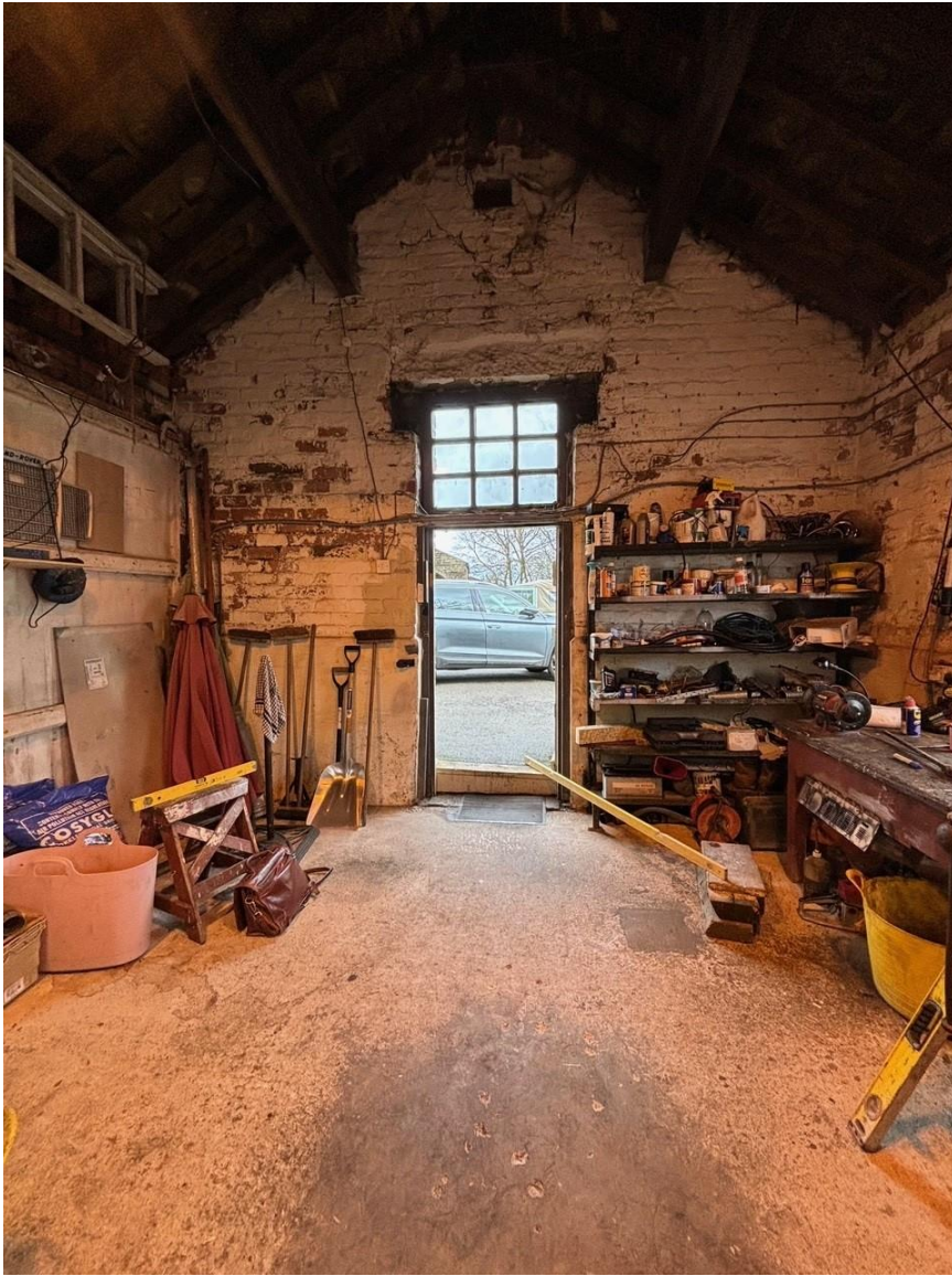
Internal view of the door
