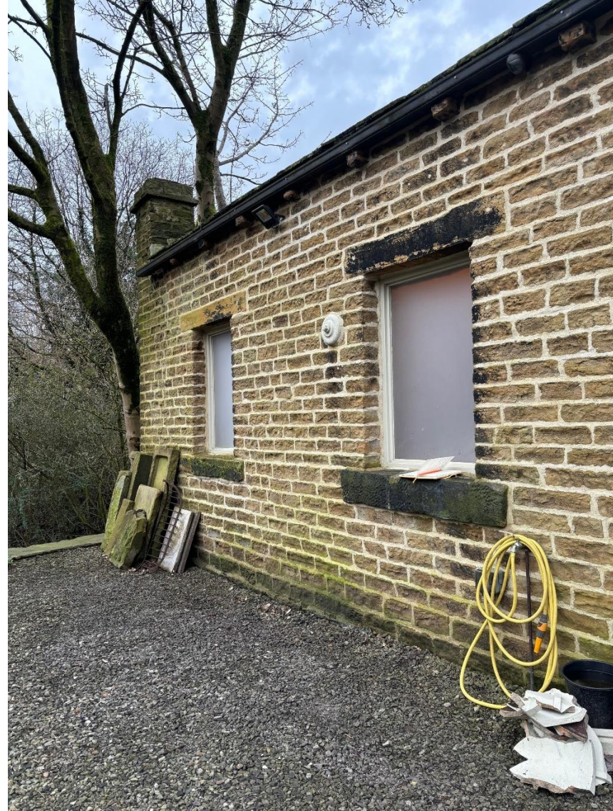
Southeast elevation / rear of the dairy
