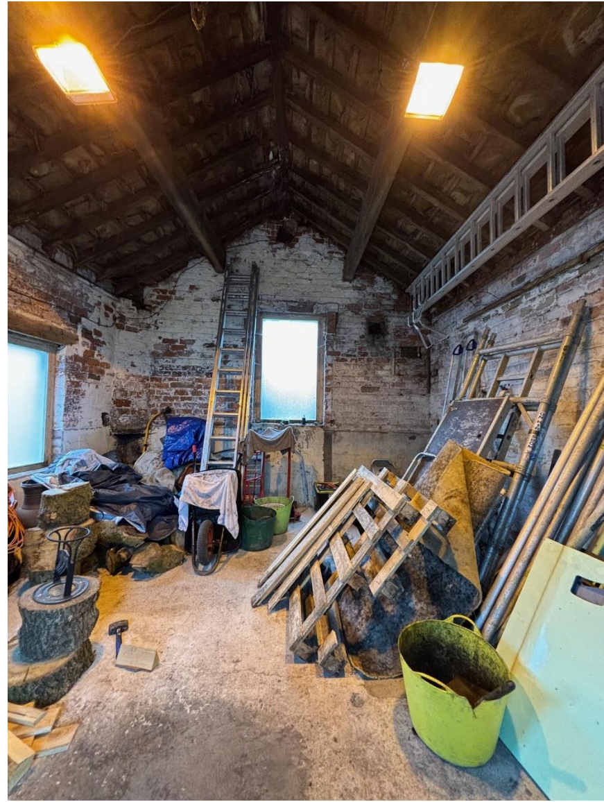
Internal view of the southwest elevation
