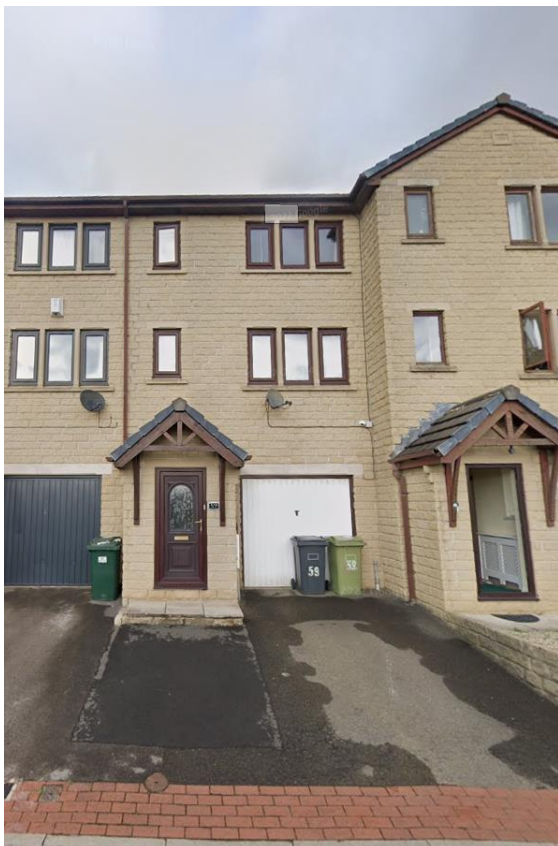
Original front elevation of 59 Cliffe Street (Plot 10) with integral garage and drive to front.
