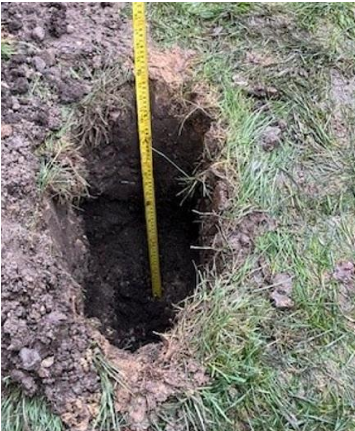
Depth check to 2ft (600mm).
