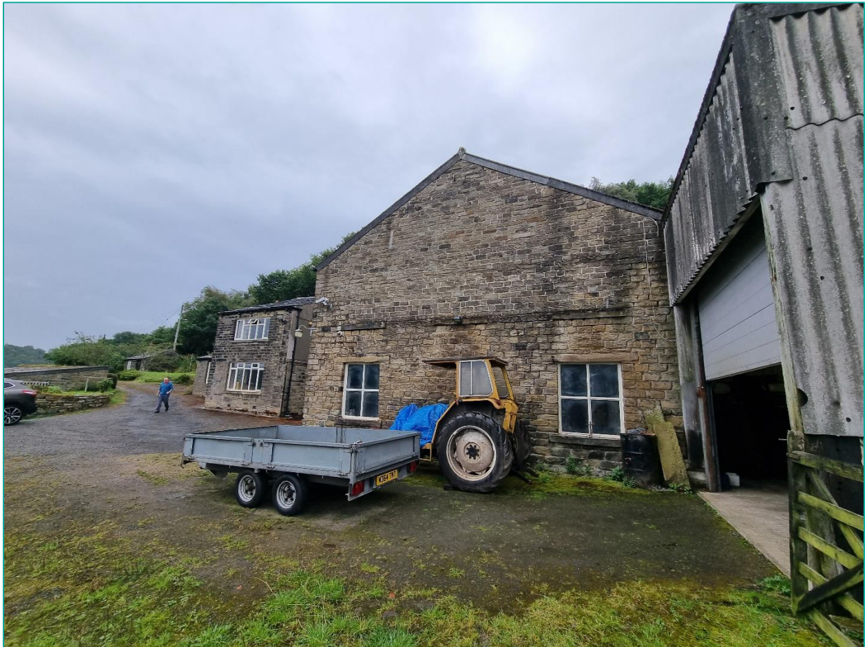
Above: Existing Barn at Granby Farm
