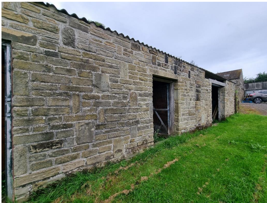
Above: Existing stables to be demolished.
