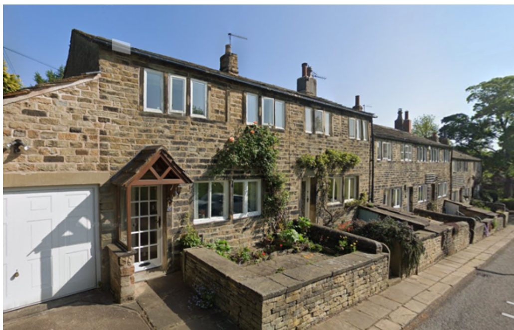
Figure 19: Bottoms terrace of listed cottages to the immediate east of the application site
