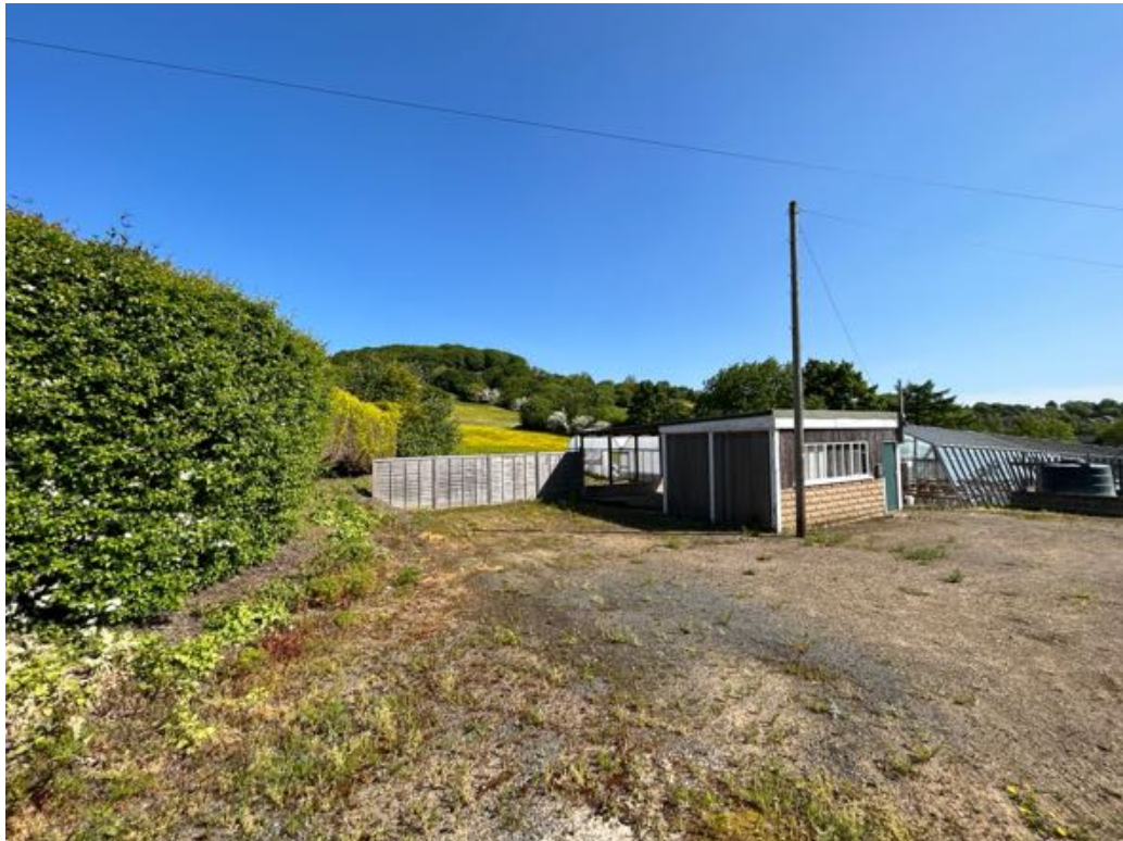
Figure 6: existing office building viewed from Lumb Lane, looking towards open countryside beyond
