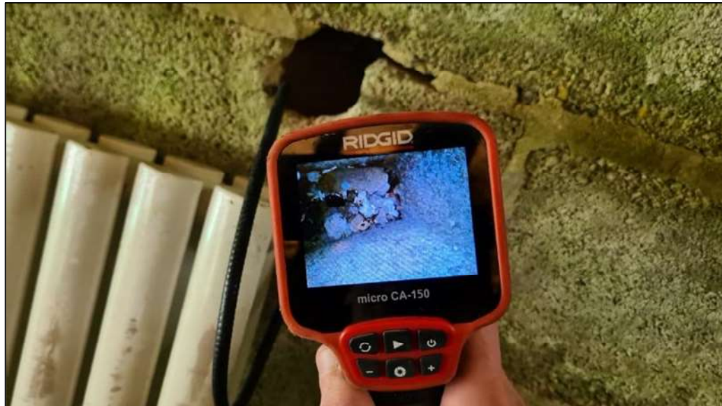
Plate 3. The hole in the hollow concrete blockwork wall being inspected
