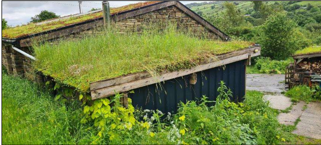
Plate 7. The composting toilet (B2) viewed from the west
