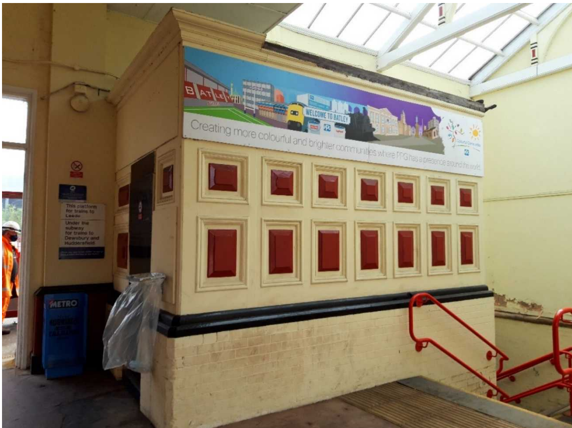
Insert 2-5 Batley Station, Interior. The stairs to the right of the photo provide access to the subway.
