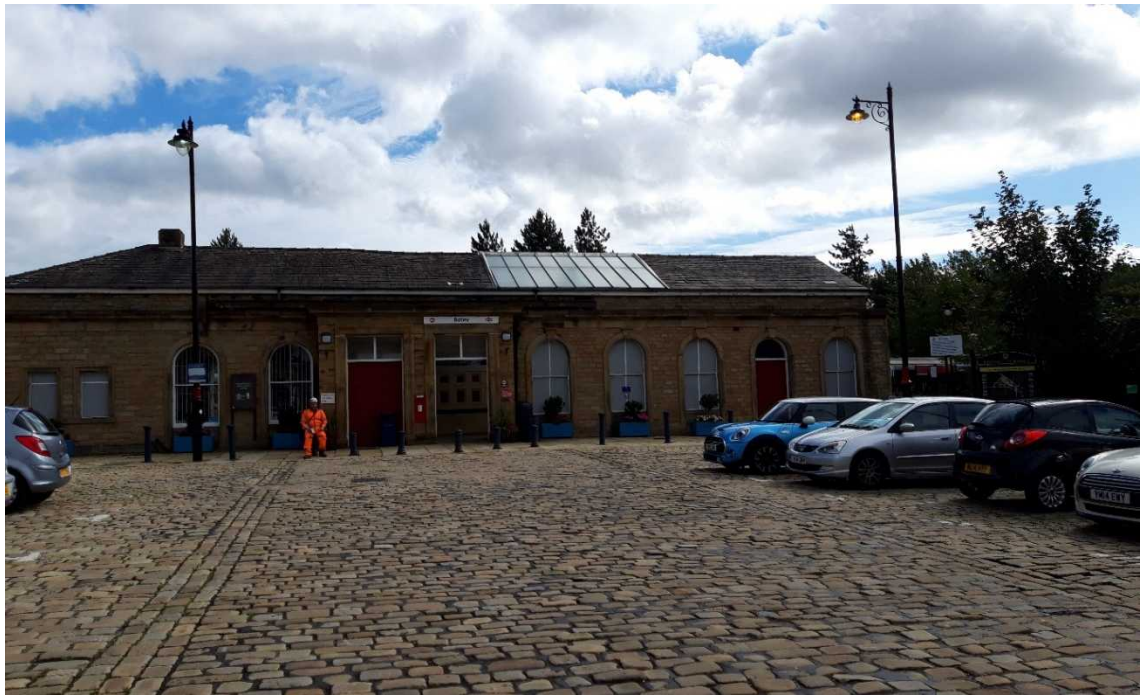
Insert 2-2 Batley Station, Western Elevation.
