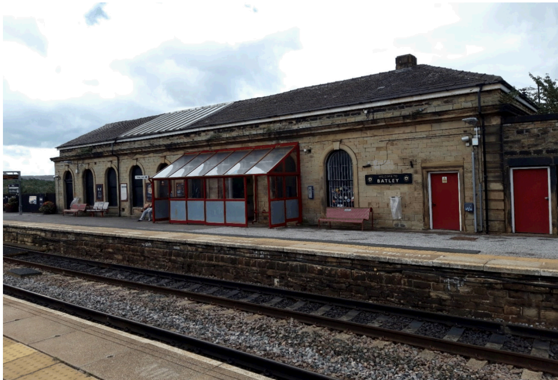
Insert 2-3 Batley Station, East Elevation.
