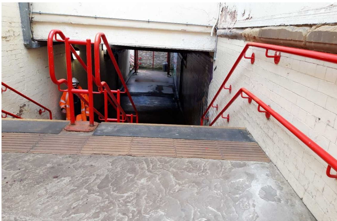
Insert 2-6 Batley Station Subway from inside the Station building.
