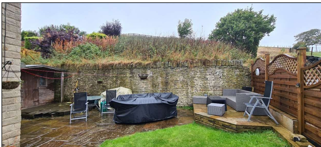
Plate 6. The lawn, patio and retaining wall at the northern end of the dwelling (2022)
