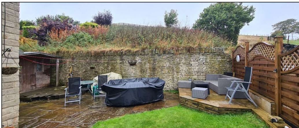
Plate 2. The retaining wall separating the existing garden from the rest of the site
