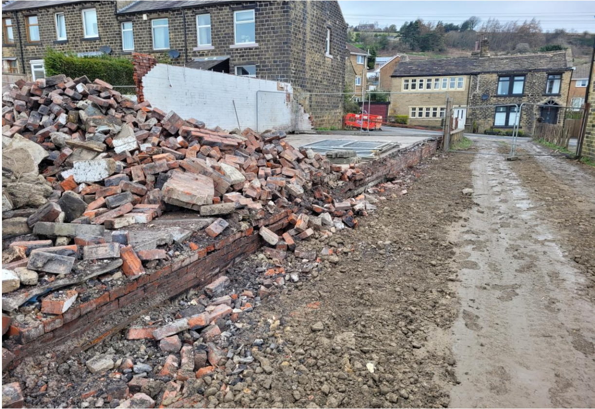
Plate 1 – Slab remaining in area of POS
