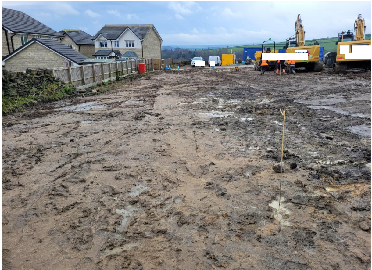
Plate 3 – Area of former ACMs reduced to natural ground (looking south)
