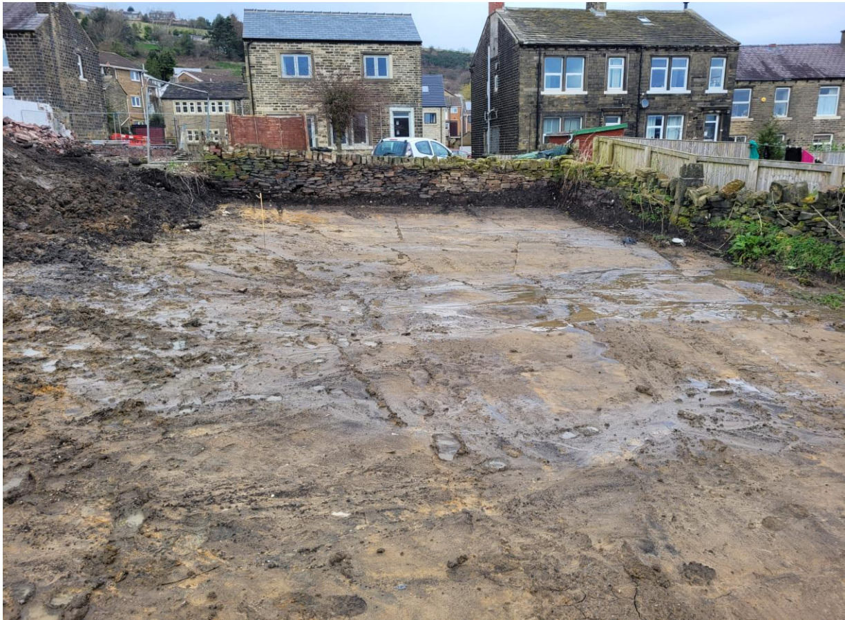
Plate 2 – Area of former ACMs reduced to natural ground
