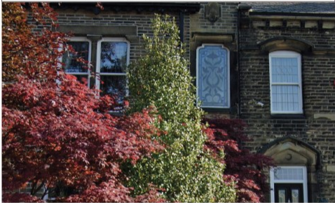
Matching Stone work to Original Dwelling
