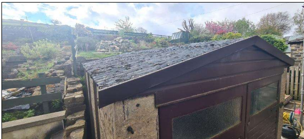
Plate 6. The garage roof viewed from the northeast
