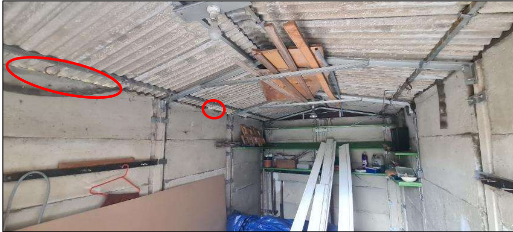
Internal inspection - garage
