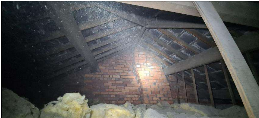
Plate 4. The roof structure
