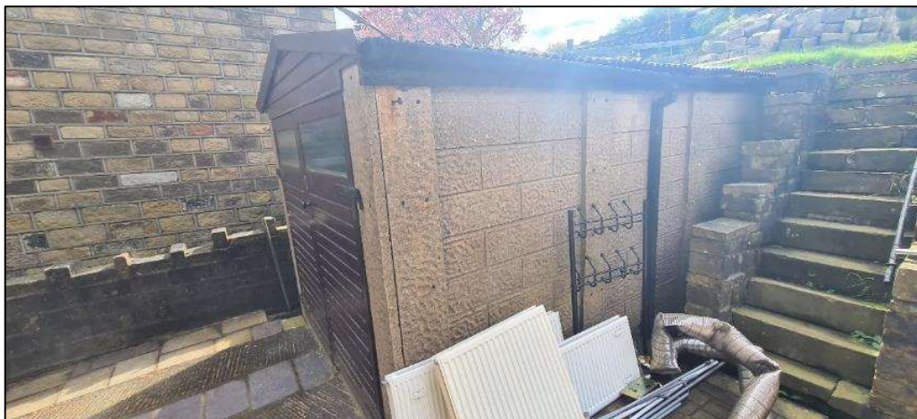
Plate 5. The garage viewed from the northwest
