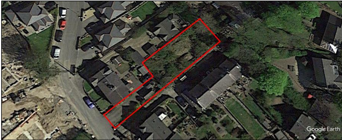
Figure 1. 2021 aerial image of site
