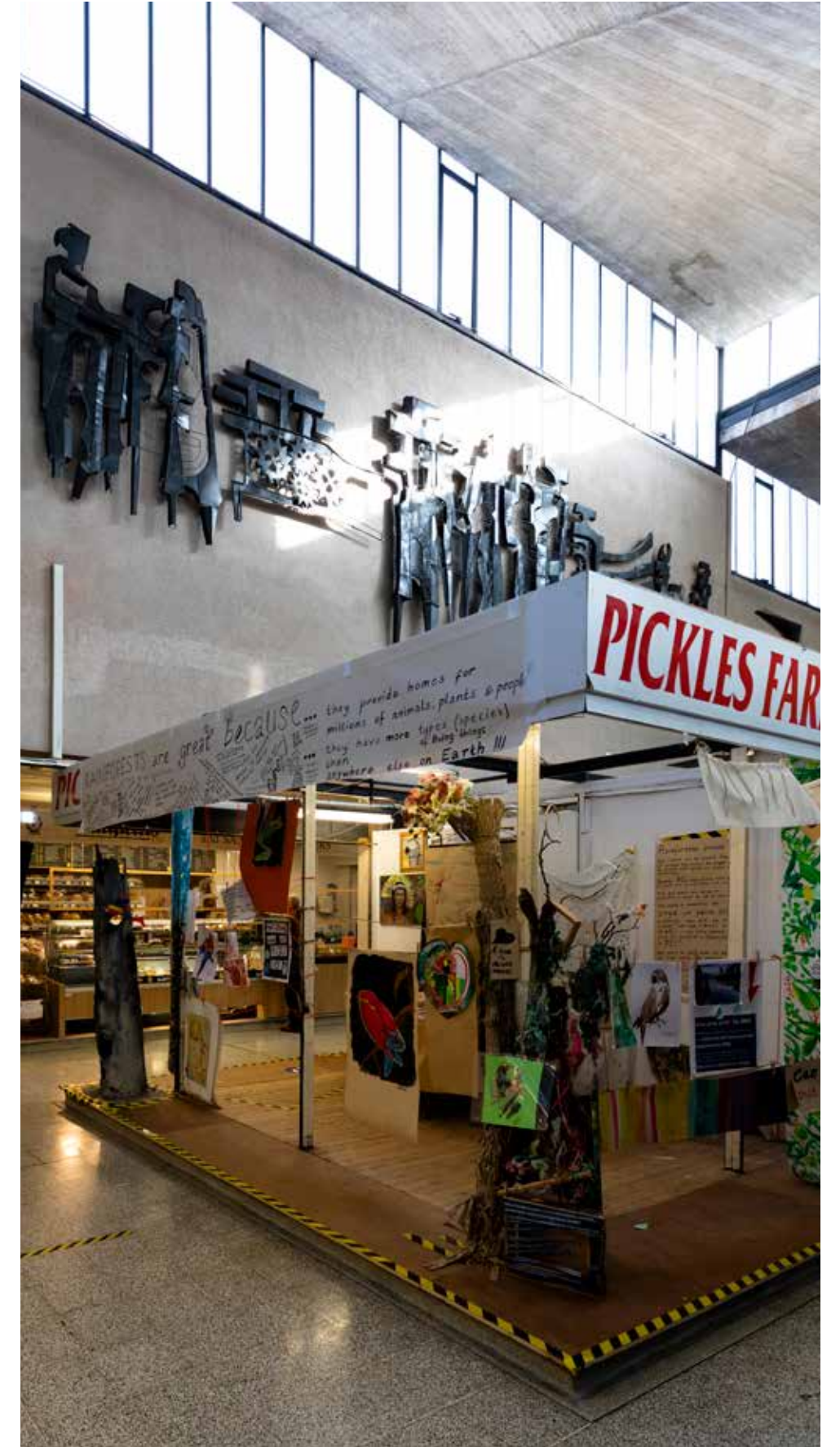
Top right: Upstand plinth of the market stall platforms visible. Some original metal market stall frames, and original terrazzo plinths with replacement terrazzo infill tiles in a number of areas
