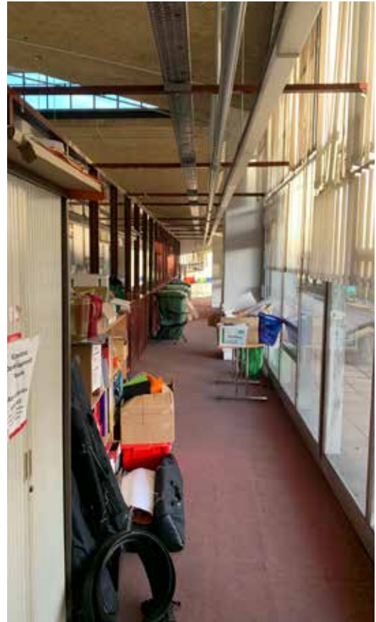
Bottom middle right: Aluminium glazing system forming print space (Rm FF-29) Top right: Over cladding and re-signage of entrances Bottom right: Aluminium glazing system as partition to original curtain glazing
