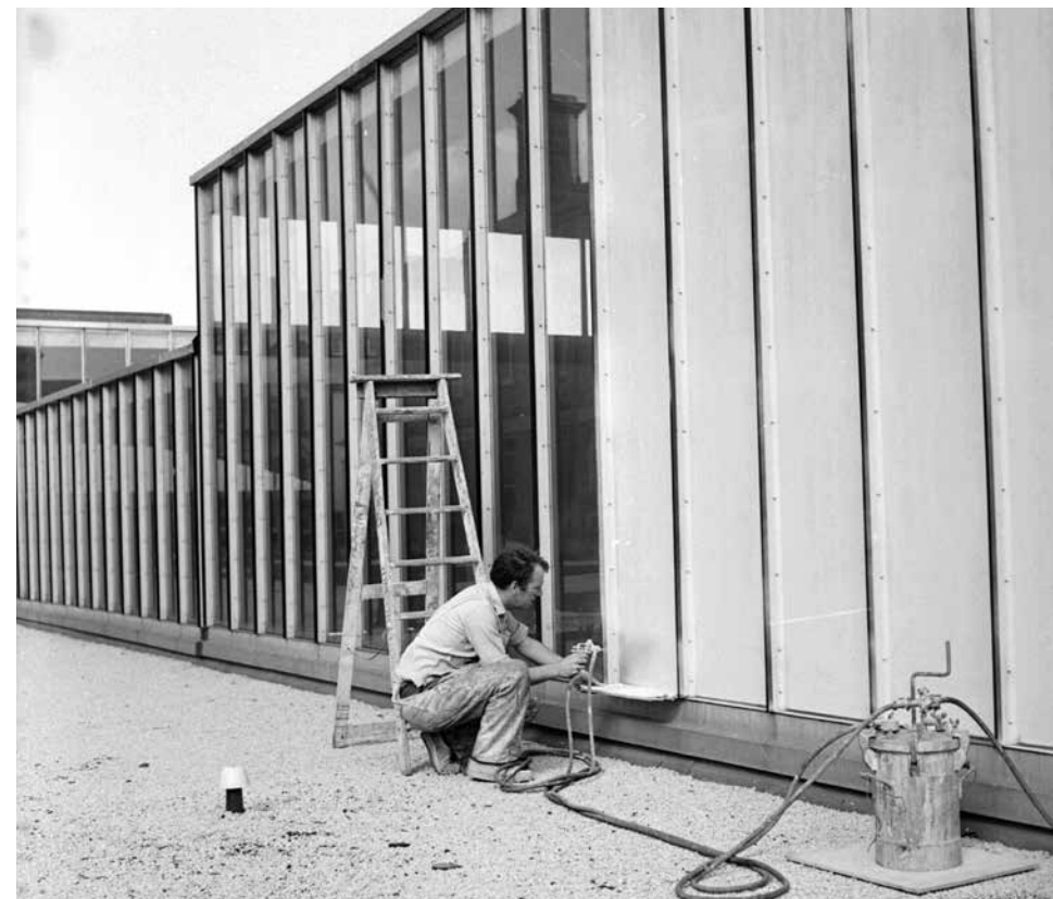
Top middle: One of the 'Articulation in Movement' ceramic sculptures now hidden behind the canopy of the trees. Bottom middle: Top hung patent glazing 1970 (Kirklees Image Archive)
