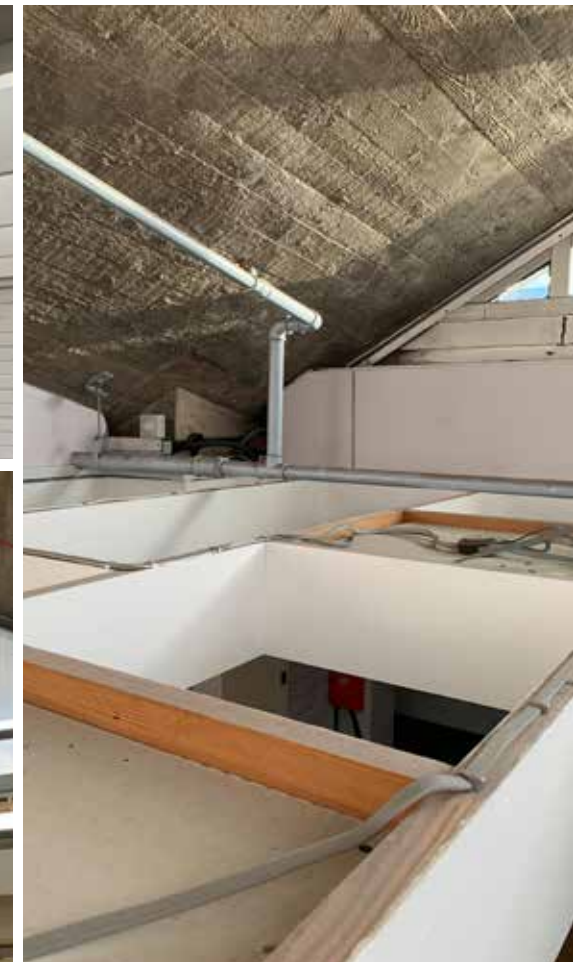
FF-21 - 27 - Above the grid, light stretching across the concrete soffit retained on show through the open ceiling grid
