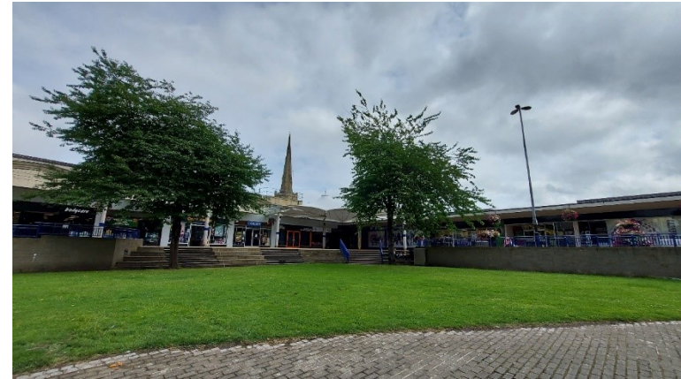
Plate 9: Views of the top of the tower and the spire from the public realm of the Piazza centre.
