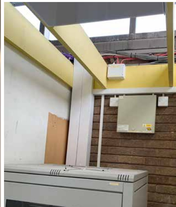
FF-08 - Server room - Grid ceiling in place
