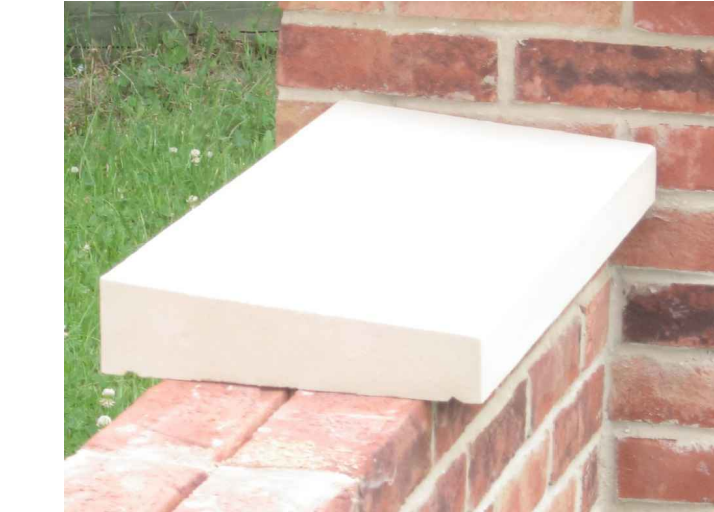
COPING STONE Once weathered coping stone to match proposed facing stonework
