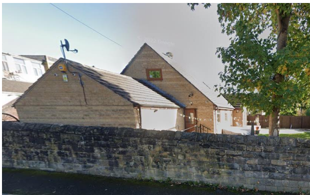
Neighbouring property adjacent to the site
