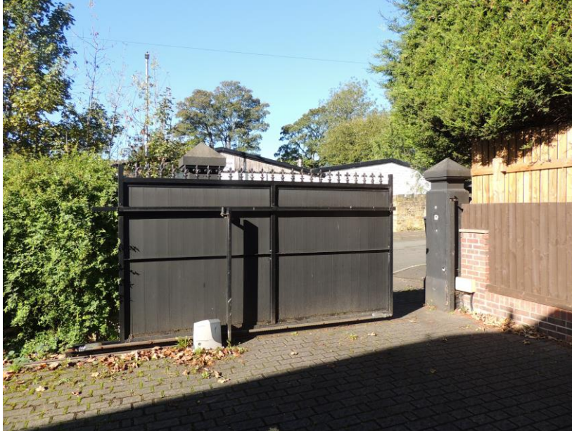
A view of the existing gated entrance providing access onto Longlands Road
