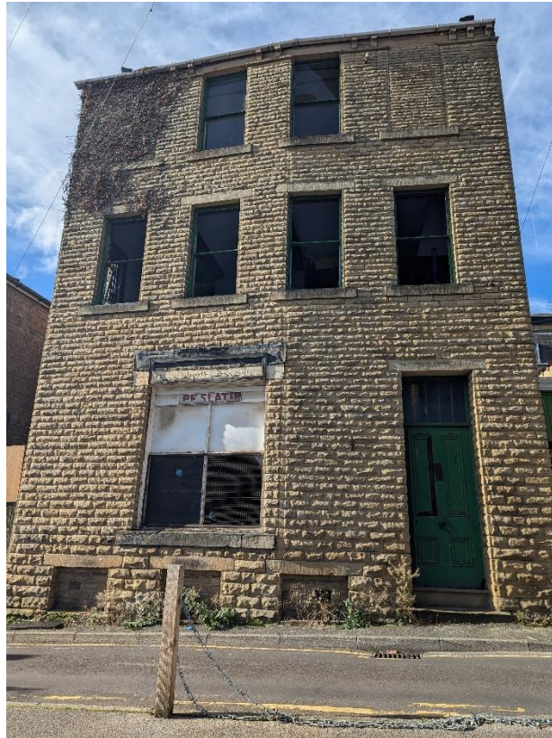
Figure 6: Facade of site
