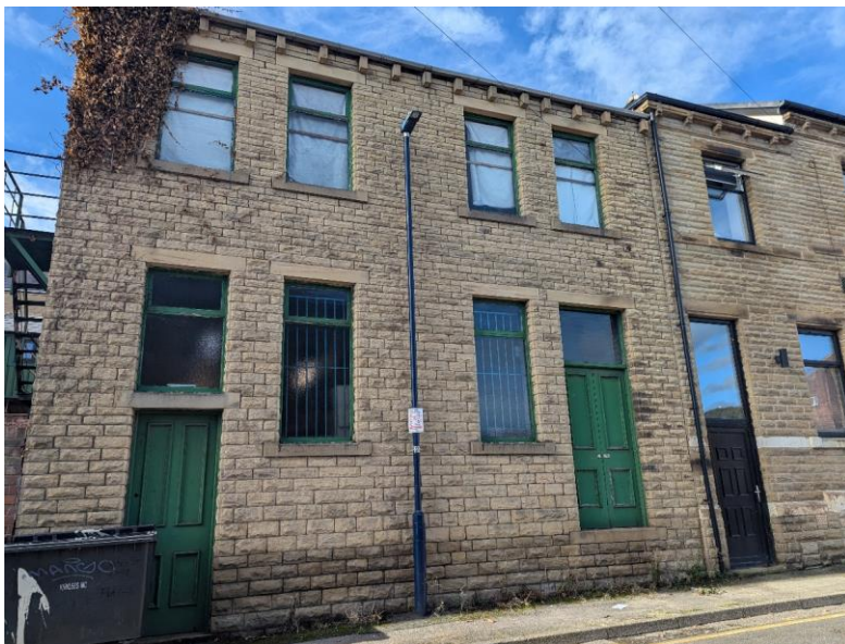
Figure 8: Industrial façade of 9 Oates Street
