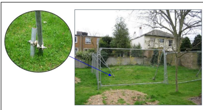
Figure A5.1: Example of mesh welded type barriers in-situ
