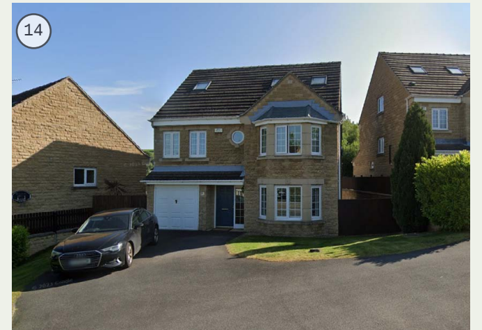
Artificial stone room in roof detached dwelling with integral garage.
