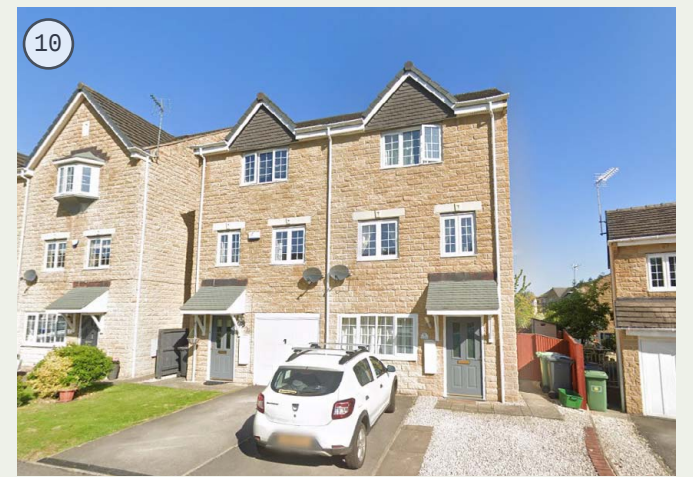
Artificial stone 3 storey semi-det dwelling with pediment feature.
