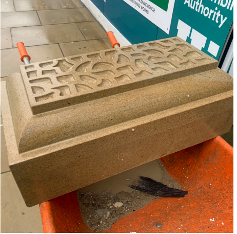
PHOTO B : Masonry repair of complete unit
