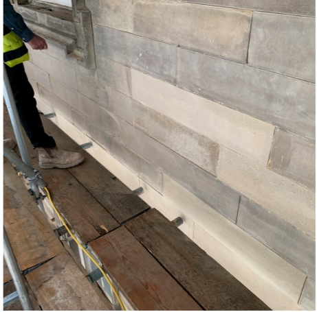
PHOTO A : Localised Masonry Repair
