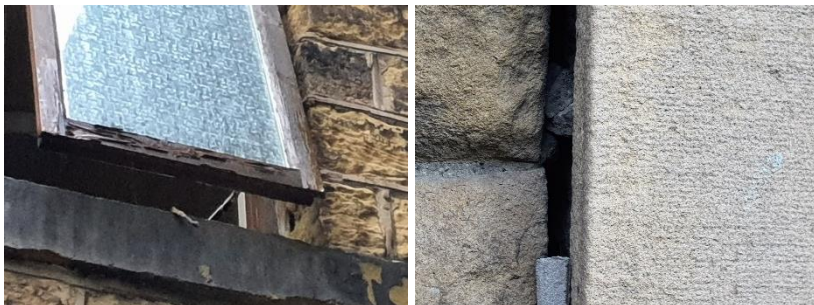
Figure 5 Showing hole to window frame (l) and door surrounding mortar (r)
